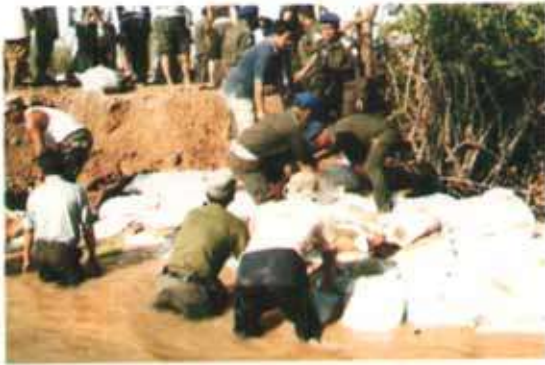
Royal Gendarmes building dams to protect against flooding in Kampong Cham province.
