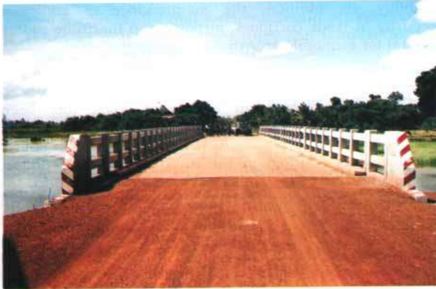
Bridges and communication routes in the countryside are built by RCAF Engineers to contribute to implementing the Royal Government's policy on poverty reduction.
